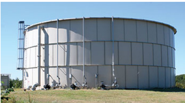
The equalization tank at Gun Barrel City's WWTP.
