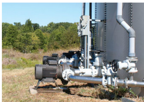
Landia's externally-mounted Airjet aeration system at Gun Barrel City's WWTP.
